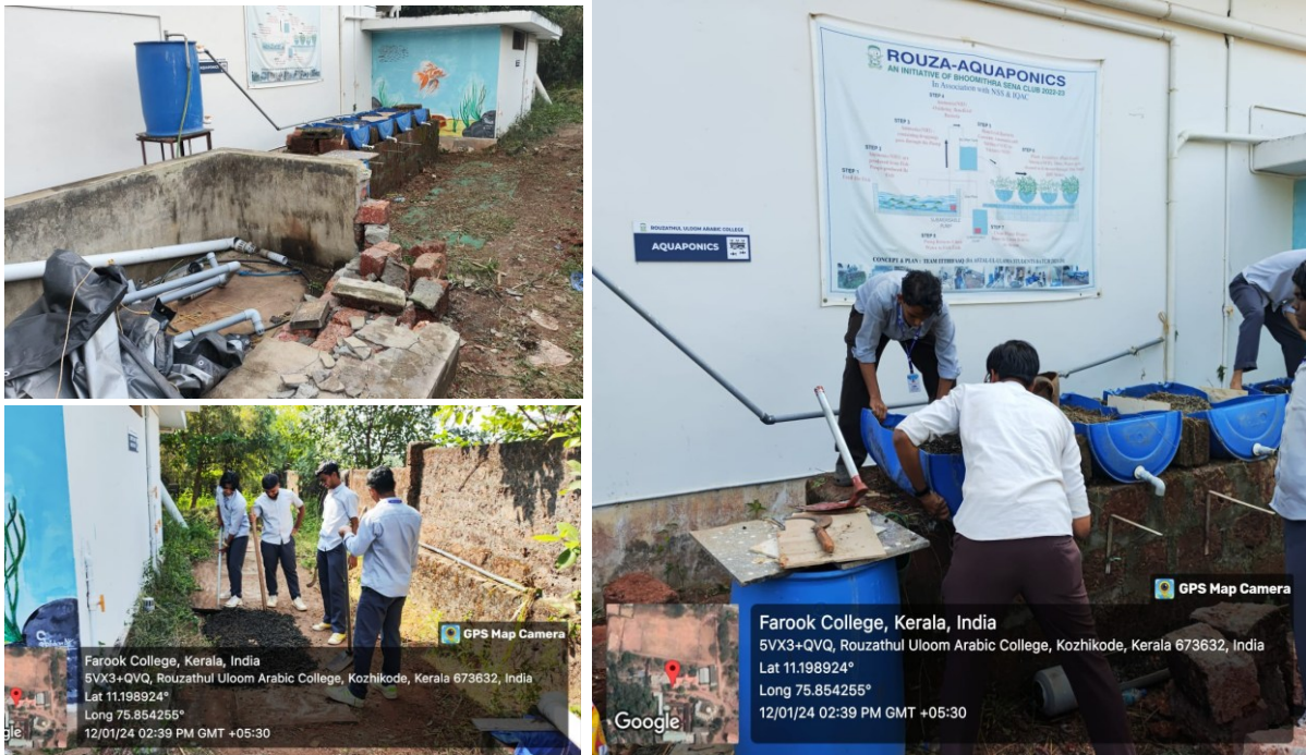
Figure 2- Bhoomitrasena Club members working on the renovation of the aquaponics plant
