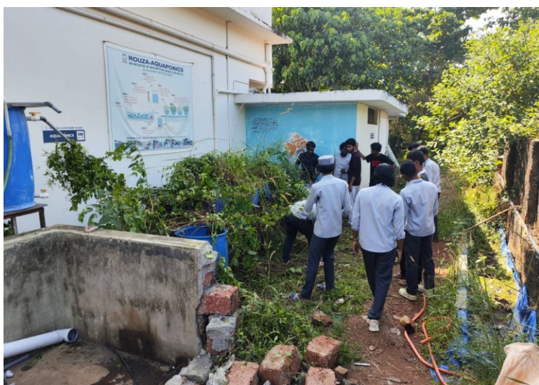
Figure 1-Club Members checking the collapsed aquaponics plant
